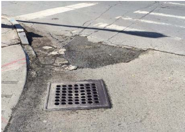
The repair 1 week later. (March 2015)
