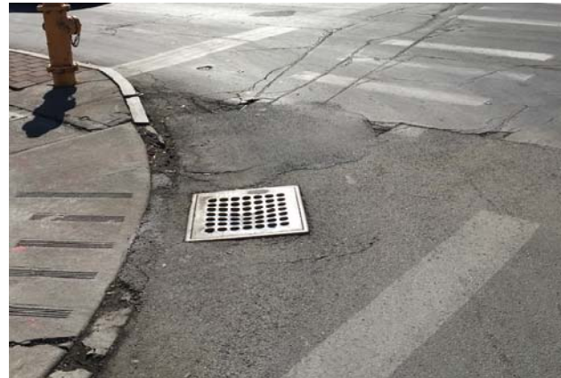
The repair 1 year later. (February 2016)
